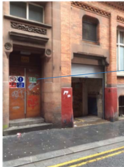
Figure 10 – concealed doorway and graffiti give this area an unsafe feel
